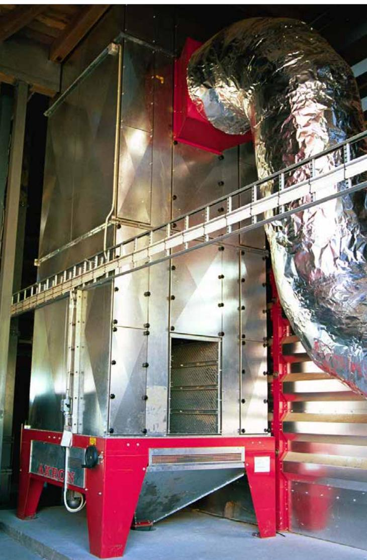
The air channel walls are designed for the lowest possible air resistance while minimising risk of grain getting stuck. Hot and cooling air intake walls are of air-sweep type while exhaust air walls have perforated slits. A common fan for both drying and cooling air minimises the risk for dust gatherings, heat leakage and condensation in the drier. The cooling zone can be adjusted for size with a simple hatch to allow for optimal drying capacity at both low and high moisture contents.
